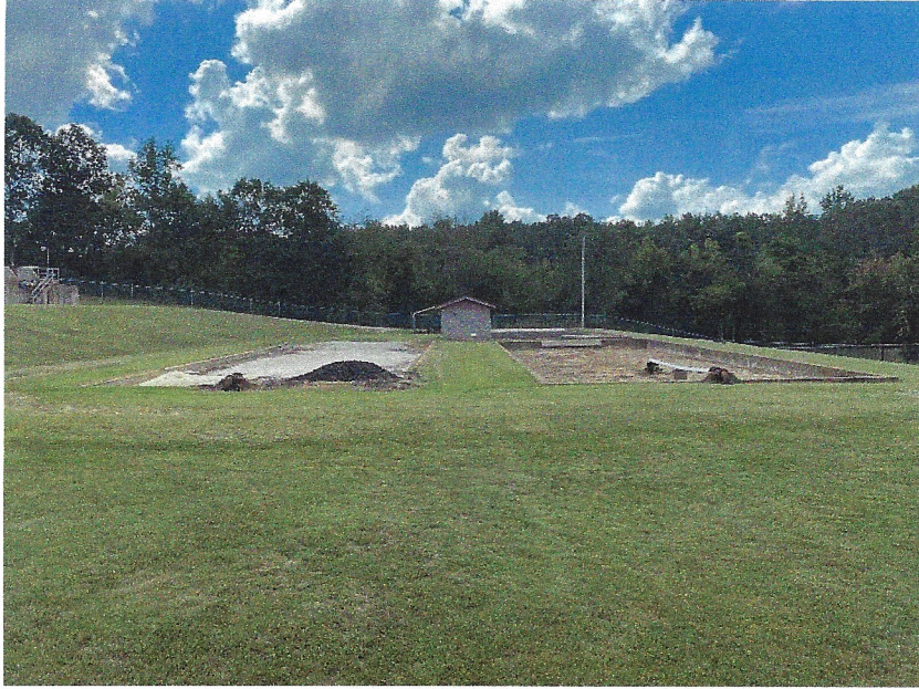
Figure 5 - Sludge Drying beds
